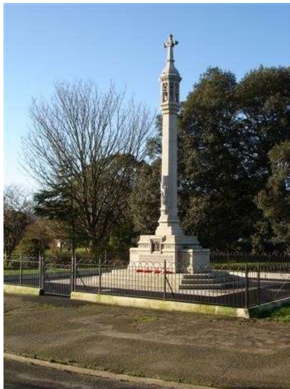
Figure 1 - picture taken before work started
