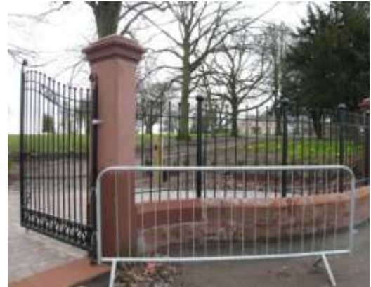
Entrance after work
