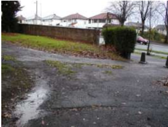
Entrance before work
