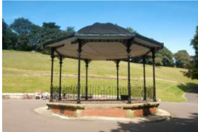
Figure 1 - picture taken before work started
